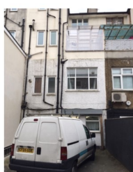
SLIA Building Rear aspect
