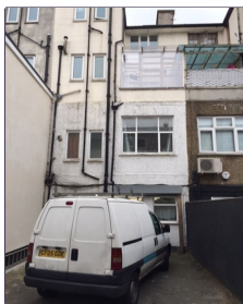
SLIA Building Rear aspect
