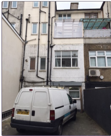
SLIA Building Rear aspect
