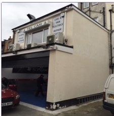
Adjacent building with rear extension
