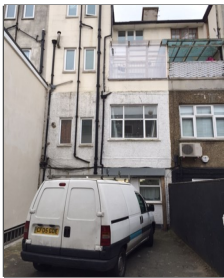
SLIA Building Rear aspect
