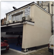
Adjacent building with rear extension
