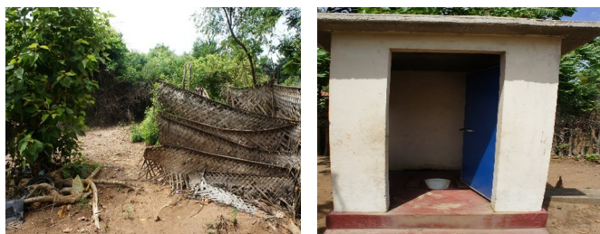
Left The family currently uses a small covering for privacy Right: One of the new SLIA / VOSD toilets
