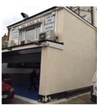
Adjacent building with rear extension
