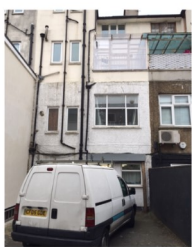
SLIA Building Rear aspect
